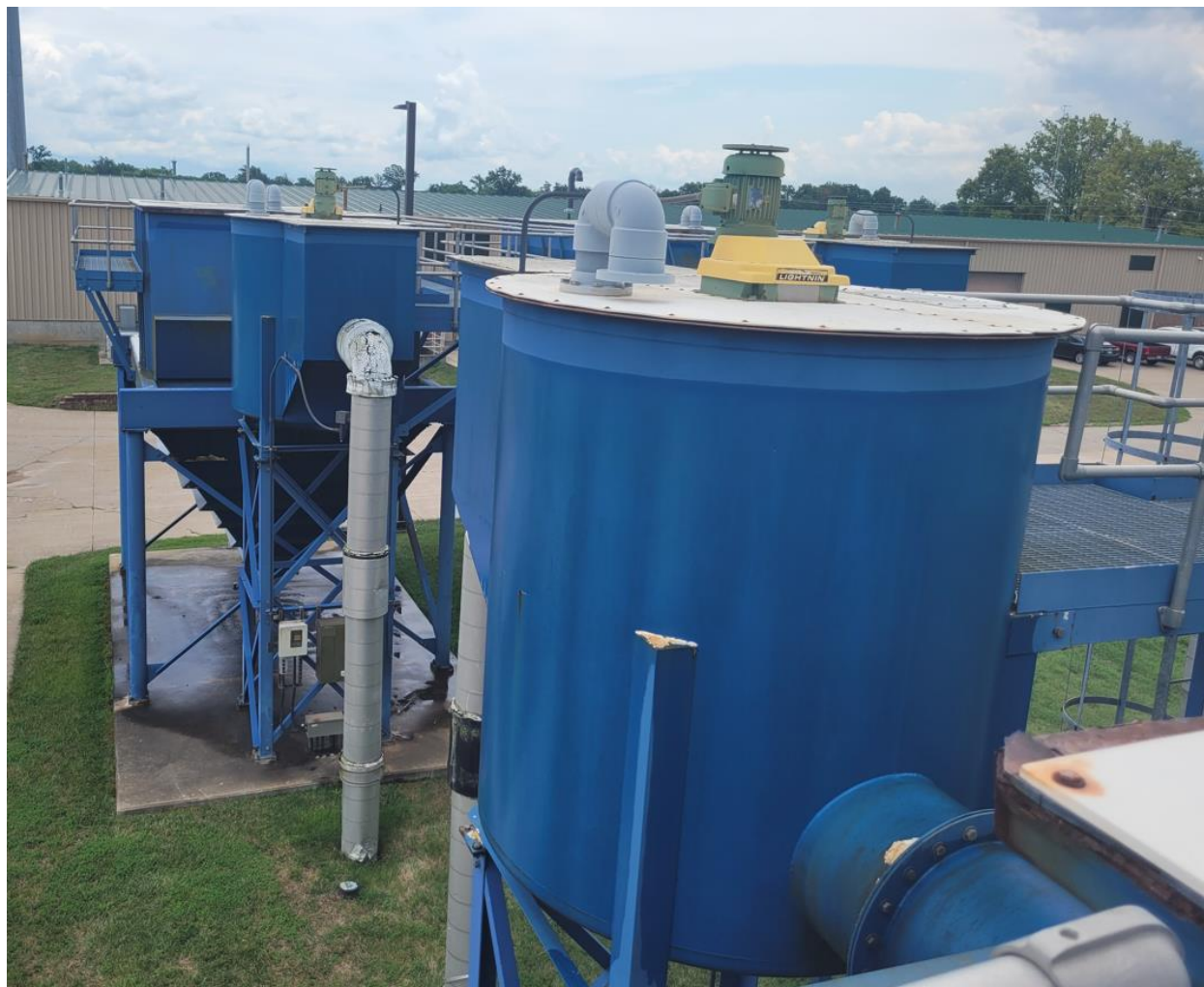
Figure 2-2: Plate Settler Units
