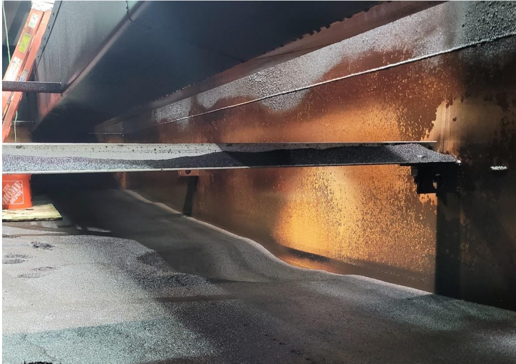
Figure 6-8: Filter 2 – Crater in Media Near Wall
