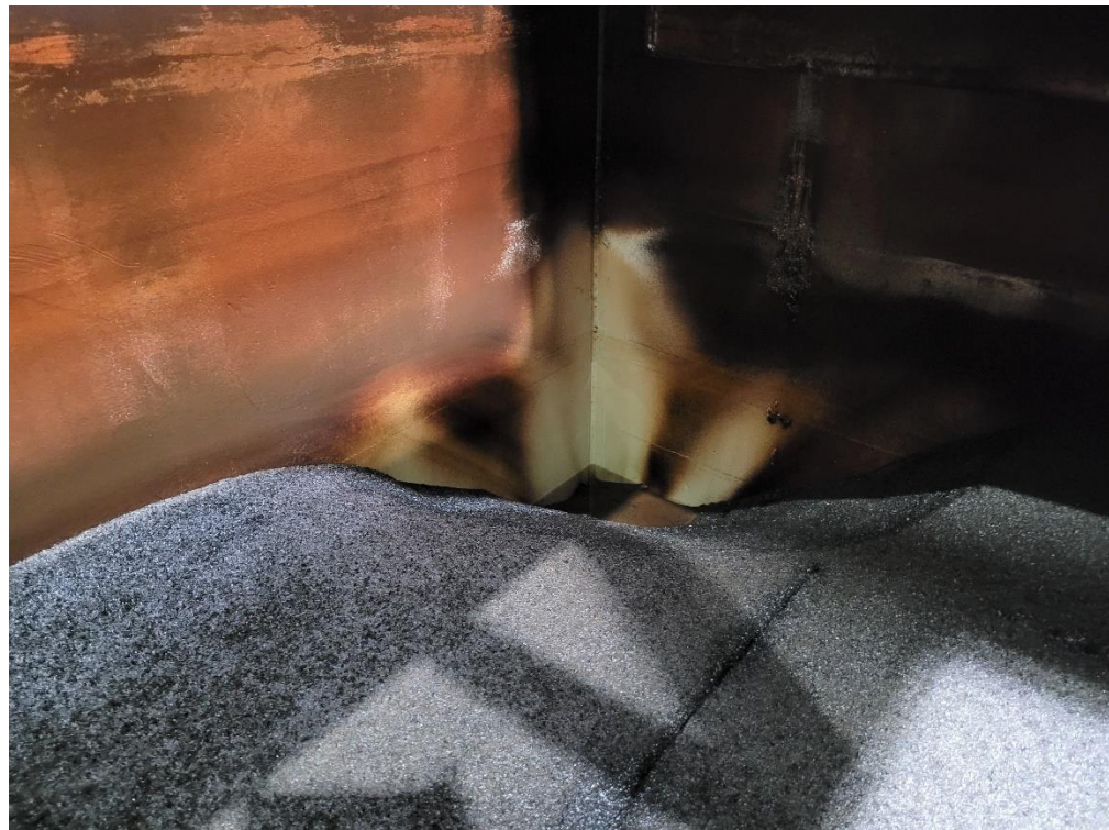
Figure 6-9: Filter 5 – Crater in Media in Corner
