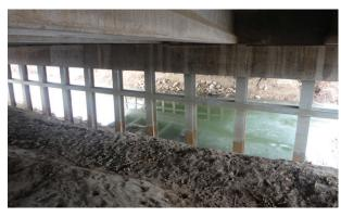
3 To accommodate the trail, regrading and retaining will be required beneath the Highway K bridge.
